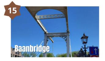
Dating from 1881, the Baanbridge is a valuable monument as a well-preserved example of a single iron drawbridge. This bridge is operated manually by means of a back chain, according to the typical Dutch design from the second half of the 19th century. As part of Edam's protected cityscape, the Baanbridge contributes to the historic character of the city.
